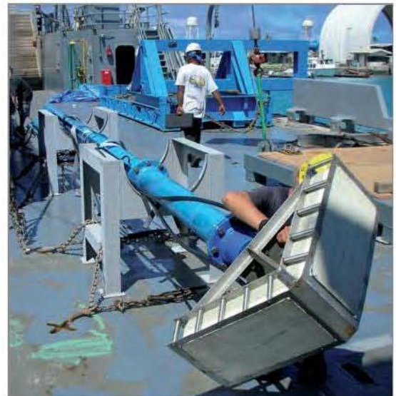
Mobile installation of transducer array
